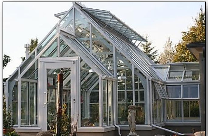
Upgrade: Entrance and Vestibule breezeway
